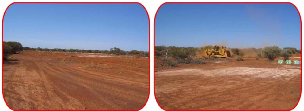
(Site clearance at Sickle Deposit underway 13 th December 2006)
